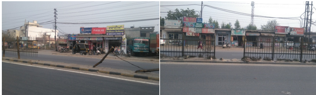
Fig. 18. Broken railing on road dividers.
