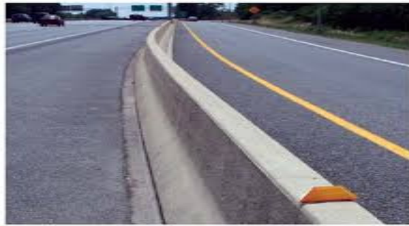
Fig. 19. Use of Concrete Barrier.
