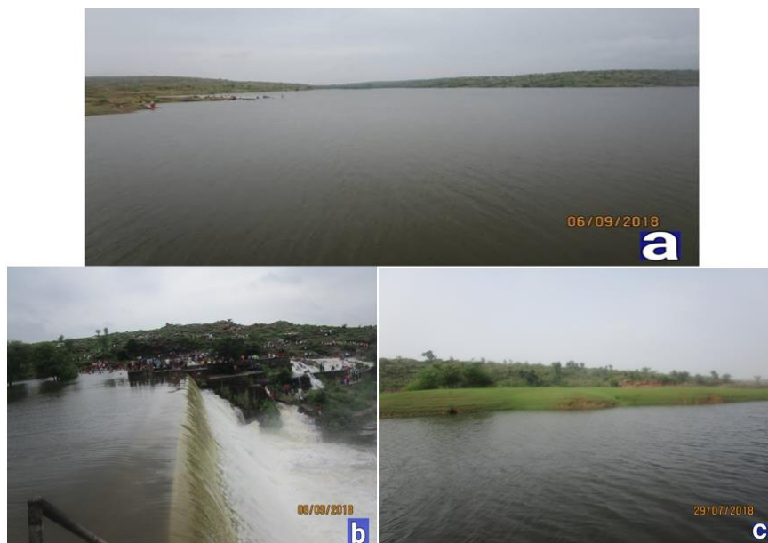
Fig. 2. Images showing actual view of Mamchari dam: Larger overview of the dam (a), Sampling Site-I (b) and Sampling Site-II (c).
