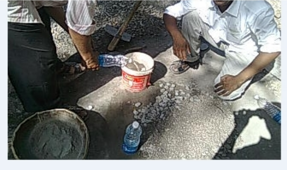
Fig. 4. Mineral water sample was being used to mixed the concrete.
