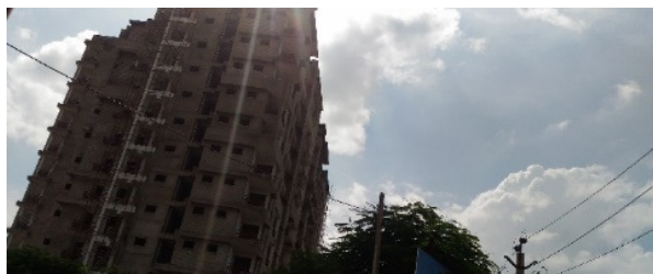
Fig. 4. High Rise Apartment to West of Kachi Basti across Amanishah Nala.
