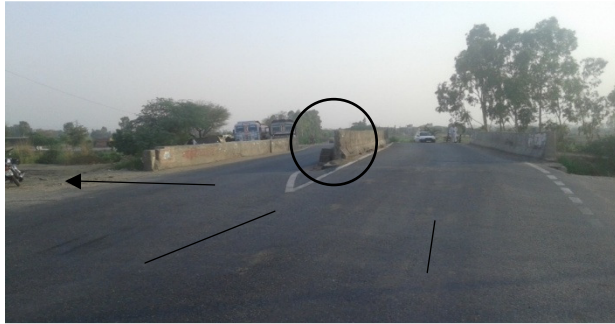
Fig. 2. Black spot on Rohat River Bridge.
