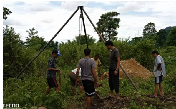
Fig. 6. Standard penetration test setup
