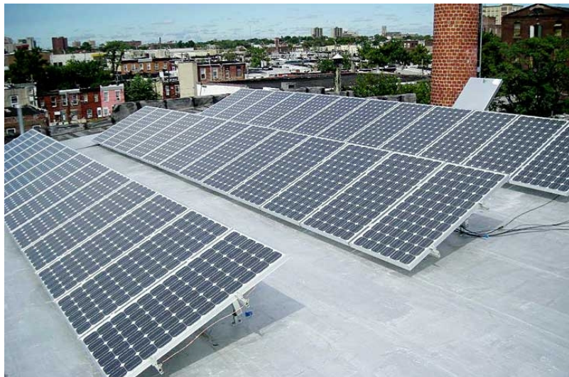
Fig. 3. Rooftop installation of Solar Panel [14].
