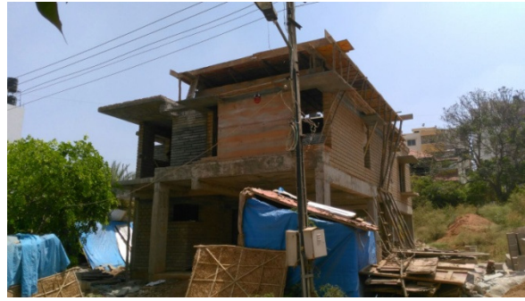
Fig. 7. A modern house with rammed earth and Jack arches.
