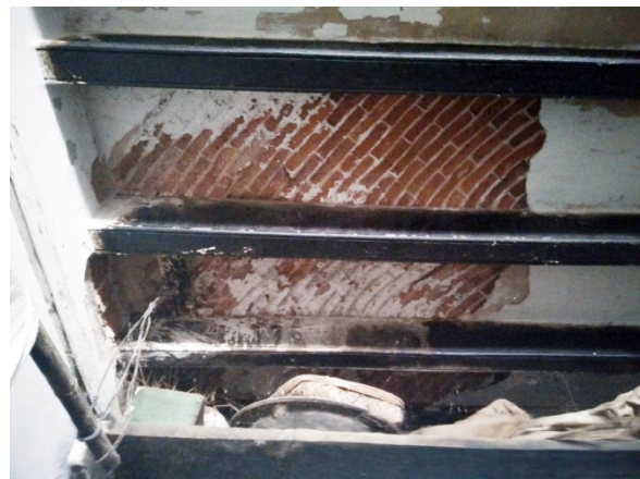
Fig. 9. Early 20th century Madras terrace exposed roof.
