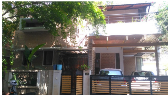
Fig. 8. A contemporary house built in Bangalore with Stabilized compressed earth blocks, Jack arches and rammed earth.
