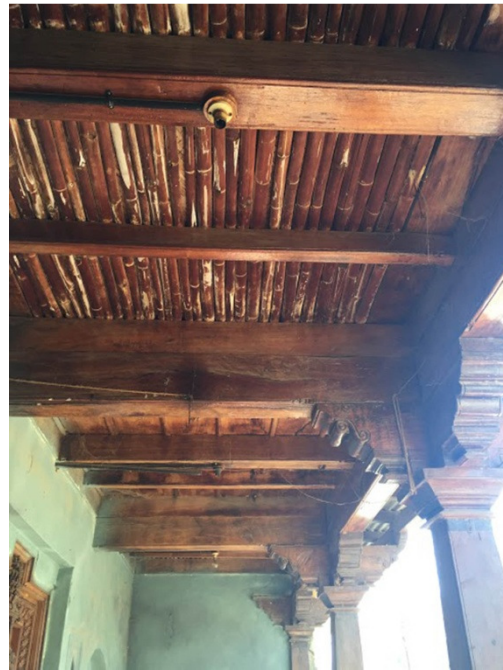
Fig. 6. Bamboo ceiling of a 'Jaggali'.
