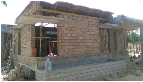
Fig. 10. A house under construction in Bangalore, designed by local architects, using Jackarche technique with steel.
