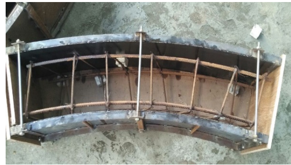
Fig. 3. Formwork with reinforcement for A4 model.
